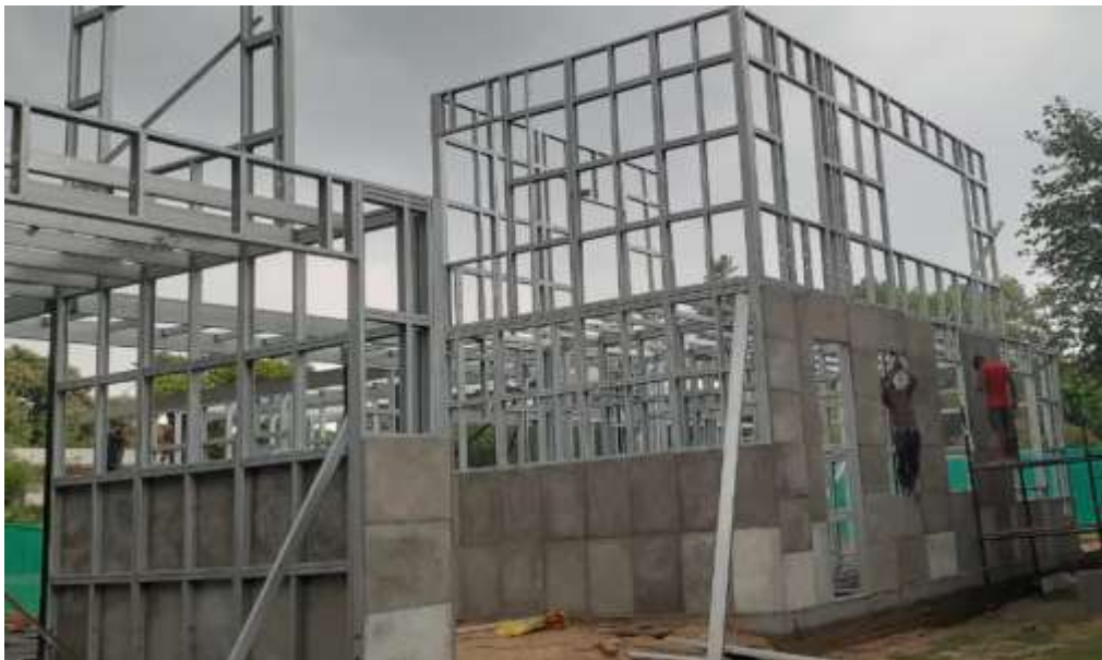
Fig. 4 Photographic view of partially completed composite building
