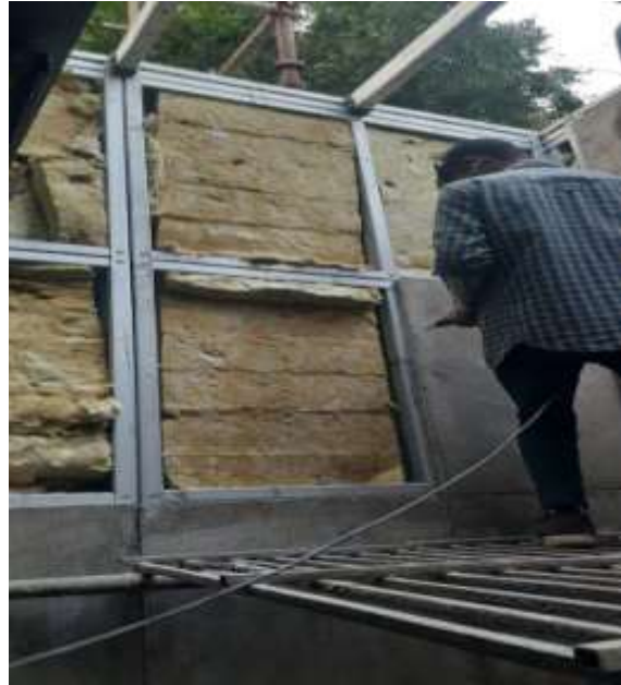
Fig. 10 Provision of Insulation
