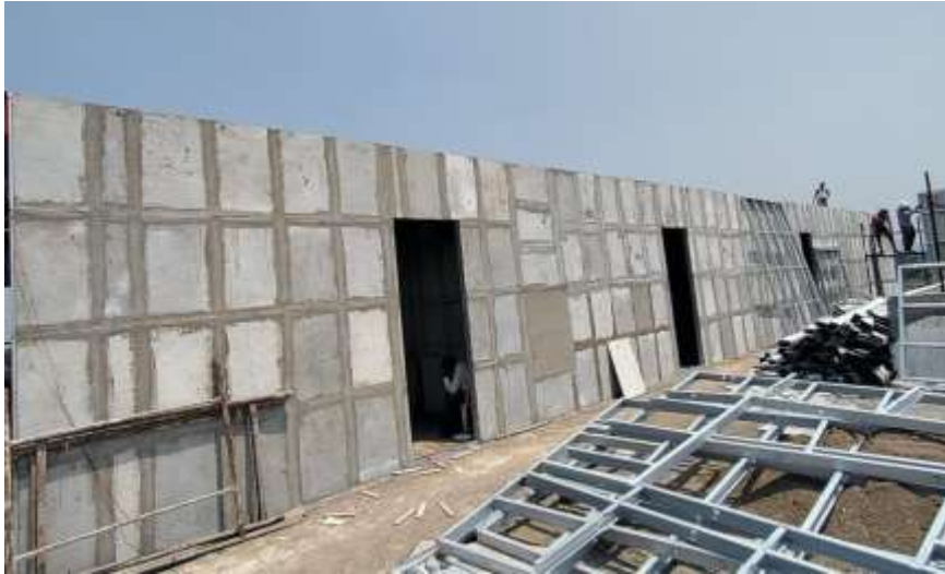
Fig. 7 Recron tape + epoxy bonder at joints for walls
