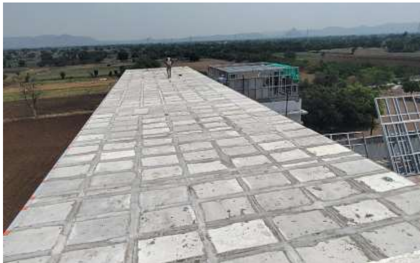
Fig. 8 Recron tape + epoxy bonder at joints for slabs
